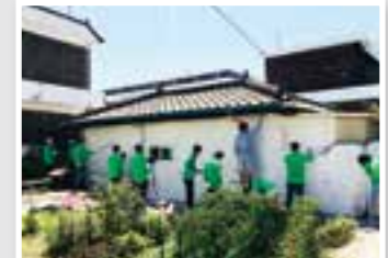
Volunteer activities of house repairs for local residents
